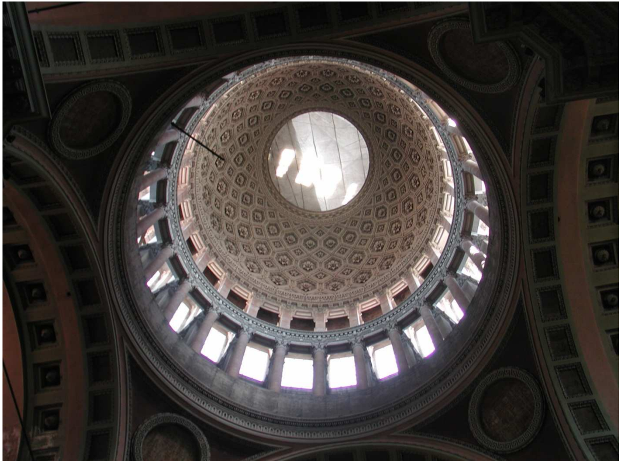
Figure 14 Dome of St. Gaudenzio (internal)
