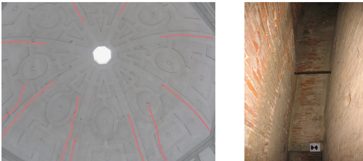
Figure 7 – On the left, View of the dome from inside the Basilica, where the first group of cracks is highlighted. On the right, Image showing the second group of cracks.
