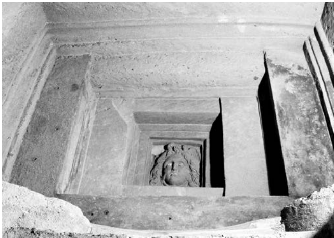
Volumni's Hipogeum, end of the III c. B.C. Perugia. Chamber with a simulated timber corbelled dome. (photo Tampone, 2010).
