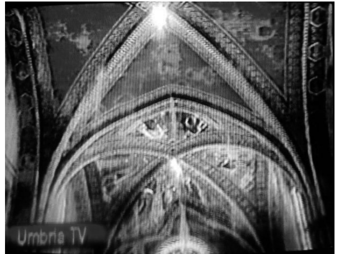
Fig. 13. The instant where the collapse began (the broken rib is visible).
