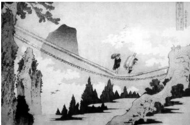
Fig. 2. A suspended bridge.
