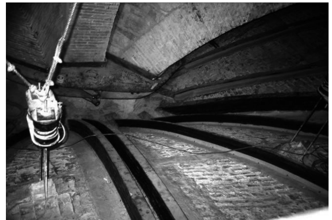
Fig. 14. The ribs on the extrados of the vaults.
