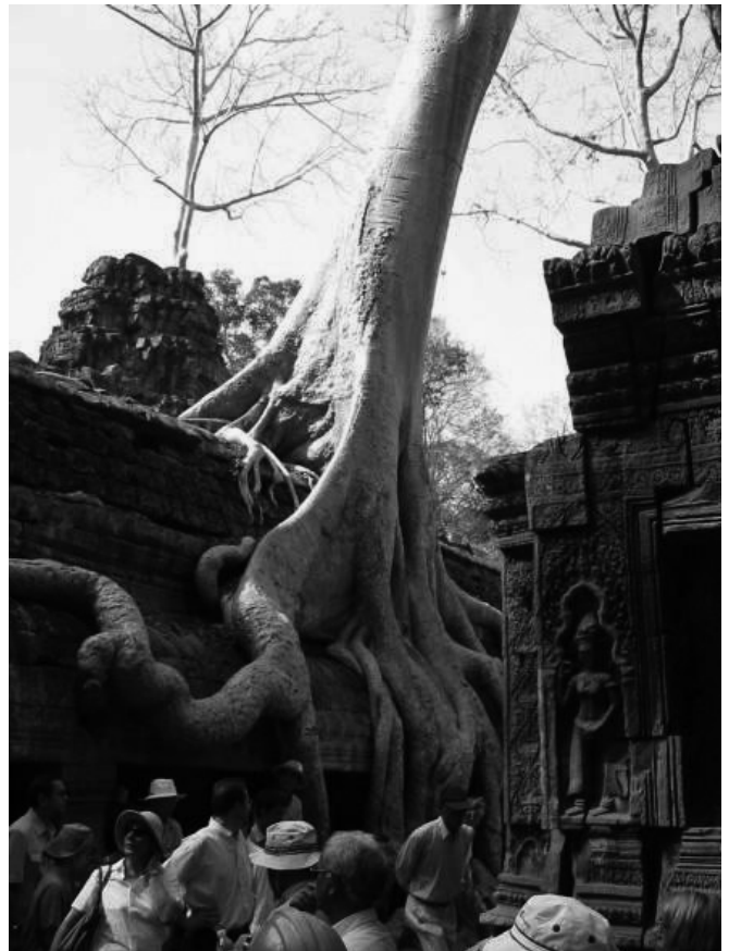
Fig. 11. The destructive effects of the roots of the trees in the Temples of Angkor.
