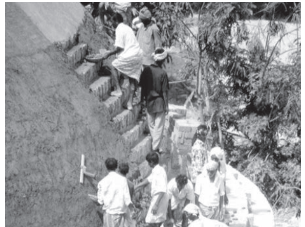
Fig. 11. Laying granite stones on the haunches.
