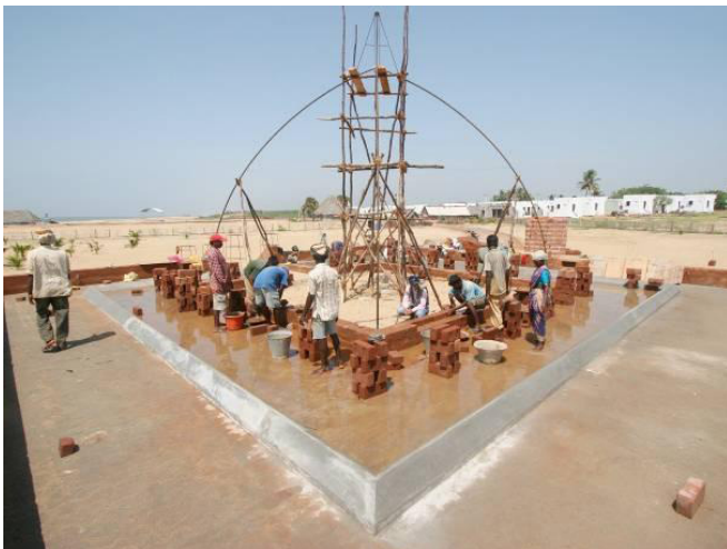
Fig. 15. Beginning the cloister dome.
