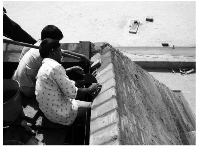
Fig. 17. Laying blocks without support.
