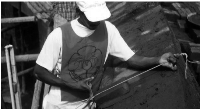
Fig. 5. Positioning a brick with the cord.
