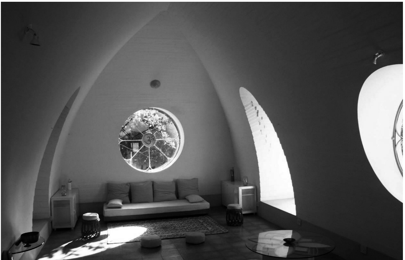
Fig. 23. Half cloister dome to close an equilateral vault.
