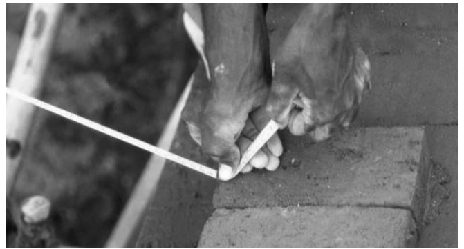
Fig. 6. Marking a 15m tape at the proper radius.
