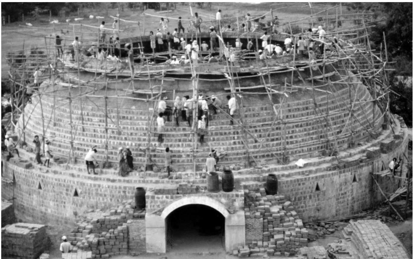
Fig. 10. Loading the haunches with granite stones.
