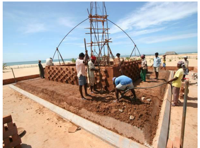
Fig. 16. Keys to link the dome with earth concrete.
