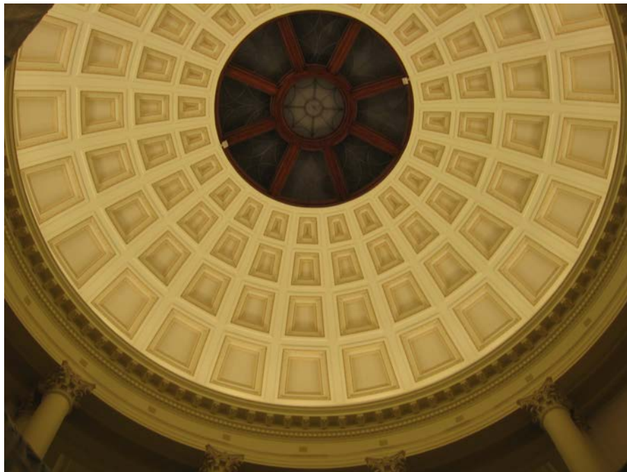
Fig. 8. Interior view of the Rotunda looking up at the restored segmented zinc-camed decorative glass laylight at the oculus of the inner dome. The original decorative paint scheme highlights the restored plaster coffered ceiling. Photo courtesy of JGWA.
