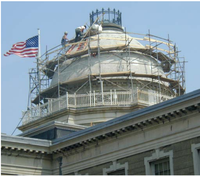
Fig. 7. Construction scaffolding surrounding the concrete dome of the Old Nassau County Courthouse, following removal of the non-original bronze coating and prior to concrete repairs. Repair mortar mock-up samples are visible on the right side of the dome, above the first stage of scaffolding. Photo courtesy of JGWA.
