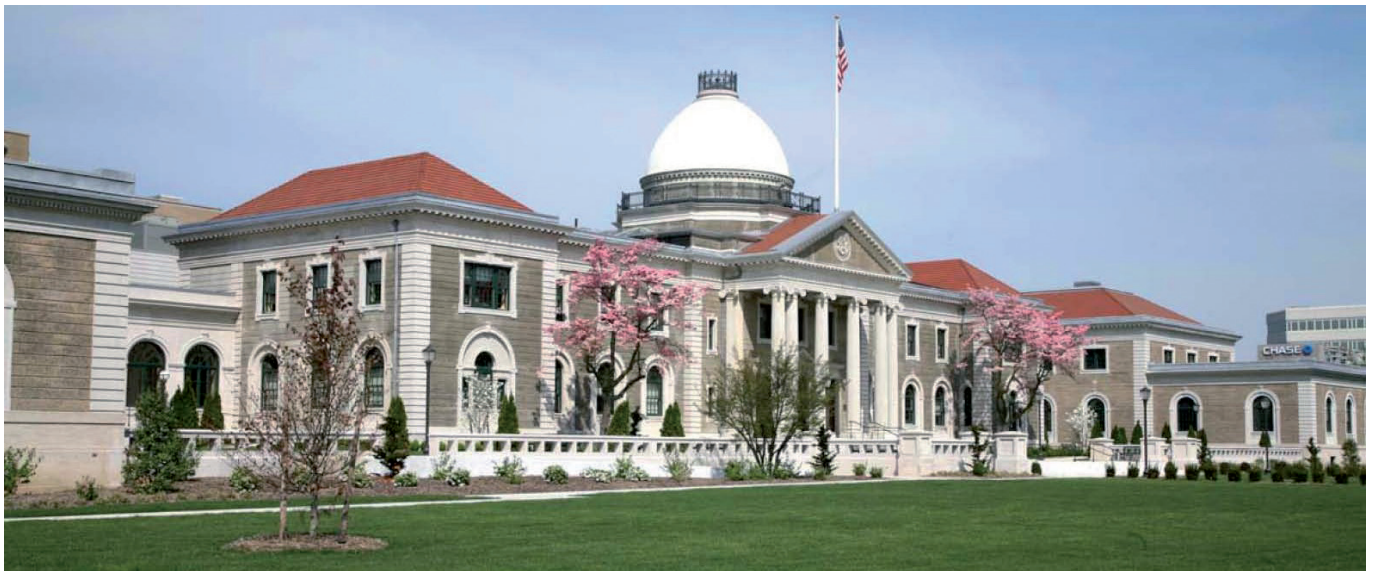
Fig. 9. The front façade of the Old Nassau County Courthouse, following a comprehensive rehabilitation of the entire building that began with the restoration of the central dome. Photo courtesy of JGWA.
