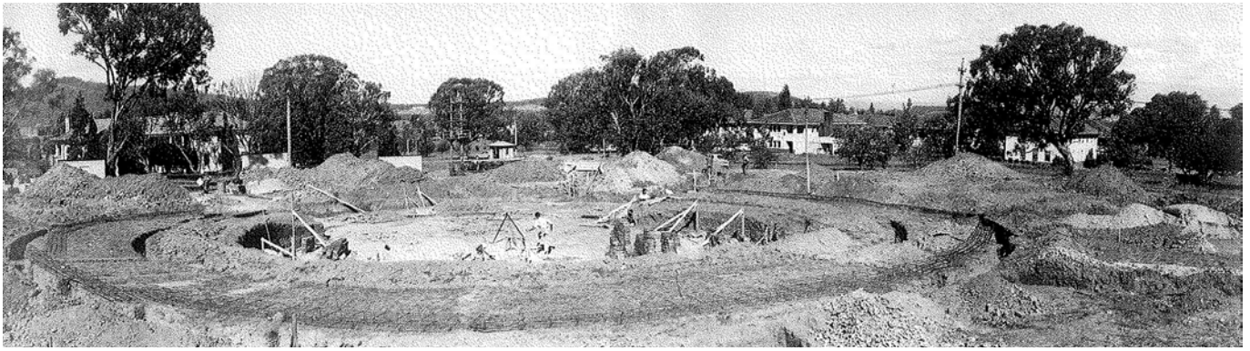
Fig. 16. Site Excavations for the Dome. Source: Roberts, A, 2010, p 71.
