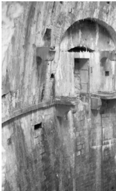
Interior view of Monte Senario's icehouse: the gallery supported by four stones corbels.
