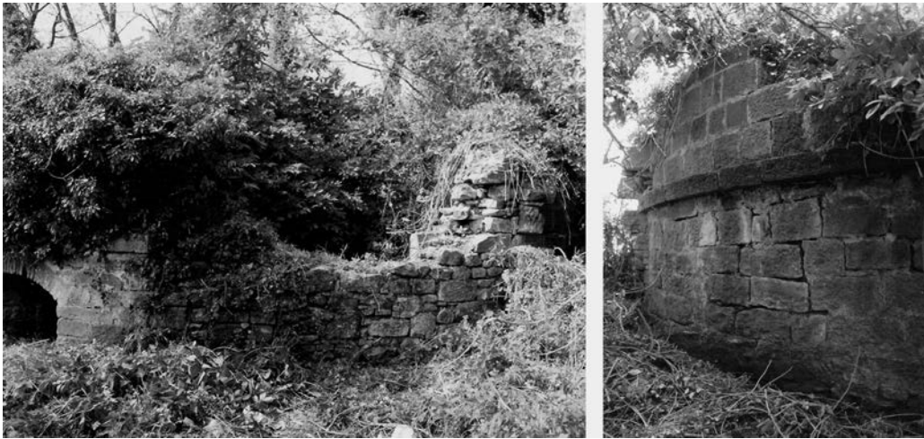
The Park of Villa Pozzolini: icehouse was made of stone and was covered with a hemispherical dome, of which only some rows of bricks remain visible.
