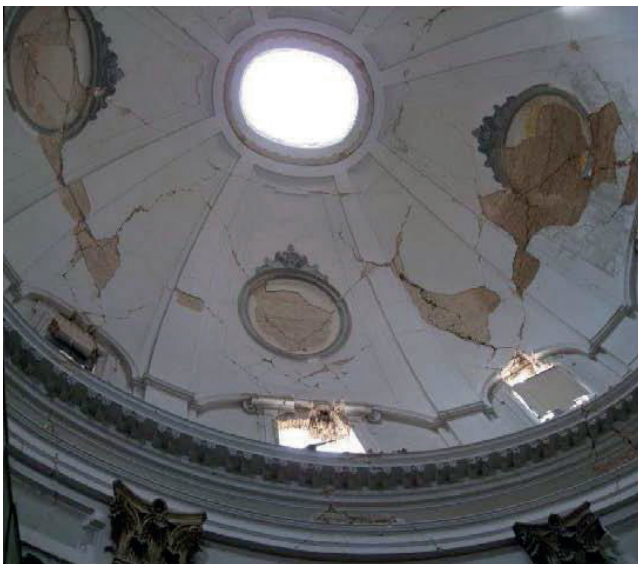
Fig. 1. Sant'Agostino dome showing the effects of the 2009 earthquake.
