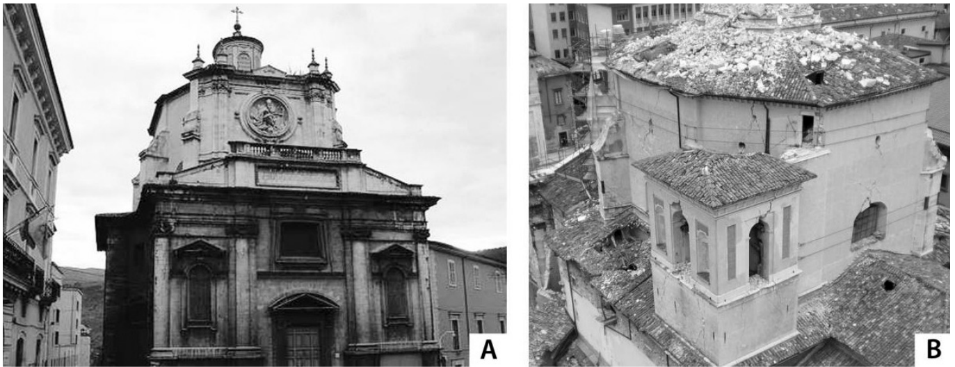
Fig. 2. S. Agostino church: (a) before earthquake, (b) after earthquake.
