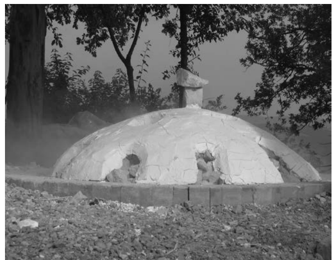
Fig. 12. Poplar boule used for the construction of the vault.
