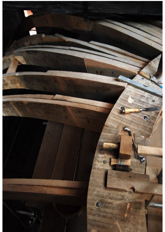
Fig. 17. The stringcourse with wooden nail.
