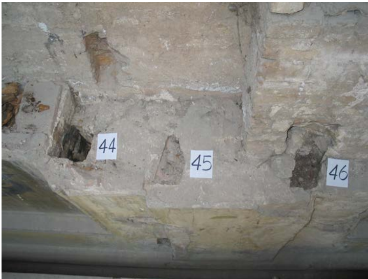
Fig. 6. The "true to life" section showing the wooden frame.
