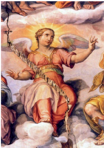
Fig. 8. Diagonal crack visible in the intrados of the internal shell (Fanelli, 2004, [6]).
