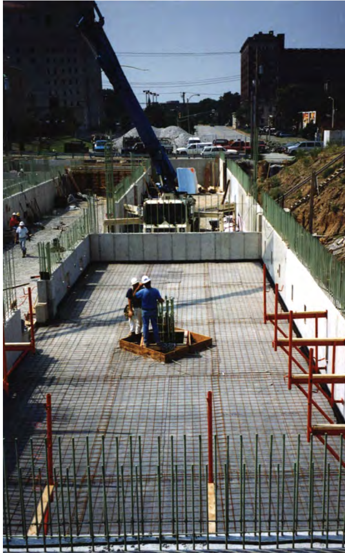
[01] Conduits for electrical work in the slab © Steve Morby
