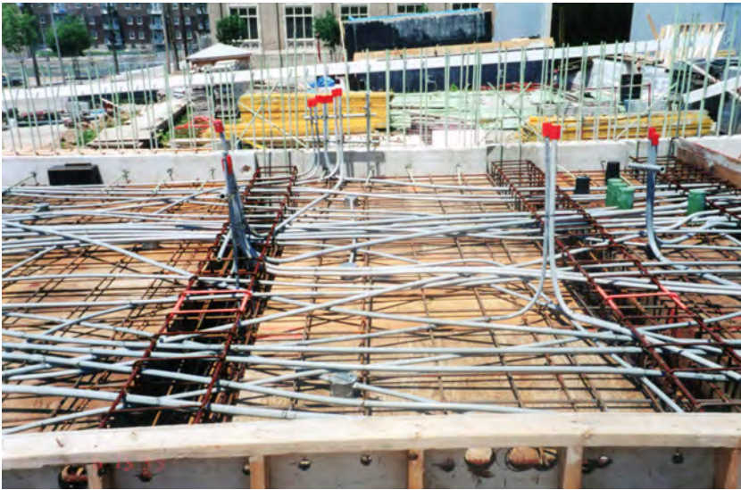
[02] Conduits for electrical work in the slab © Steve Morby
